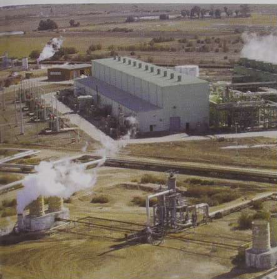
Fig. 6. Central geotermoelectrica Cerro Prieto.
